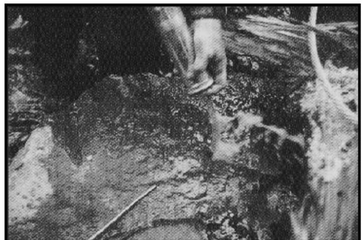
Figure 1. Boulders must be cleaned thoroughly using a wire brush and fluid sucker until the water runs clear.
